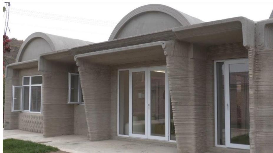
*Slika 26: House made by 3D printer*
